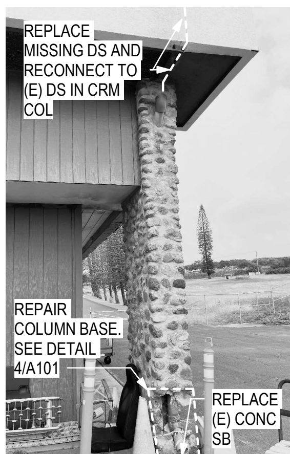
AT COLUMN GRID A1
