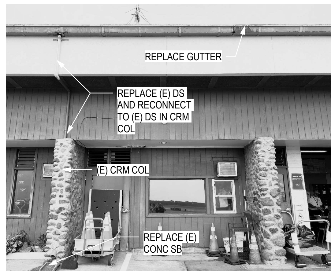
AT COLUMNS ALONG GRID A
