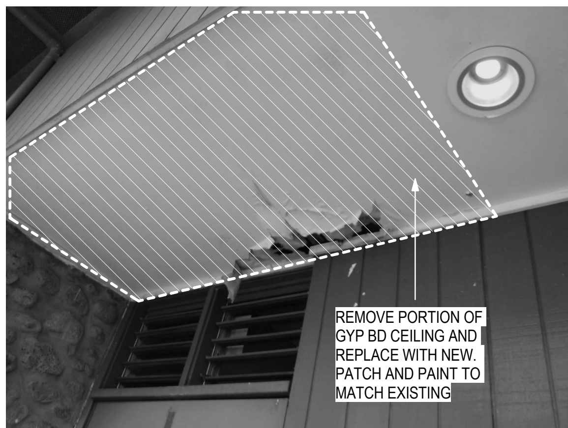
AT GRID LINE A11
