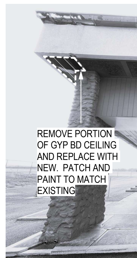
AT GRID LINE C1
