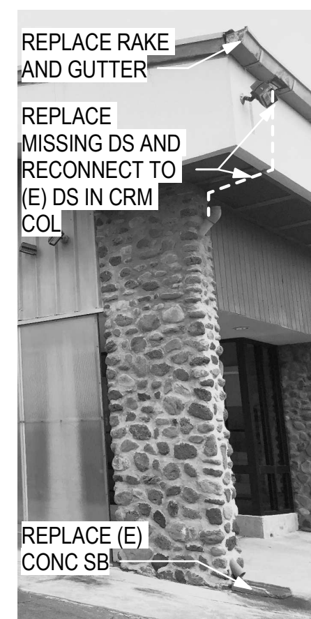
AT COLUMN GRID A15
